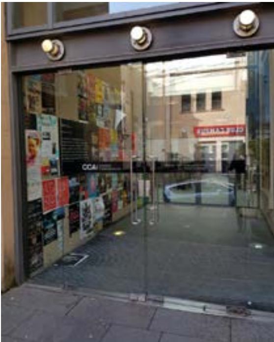
Entrance doorways from Scott Street: Exterior
