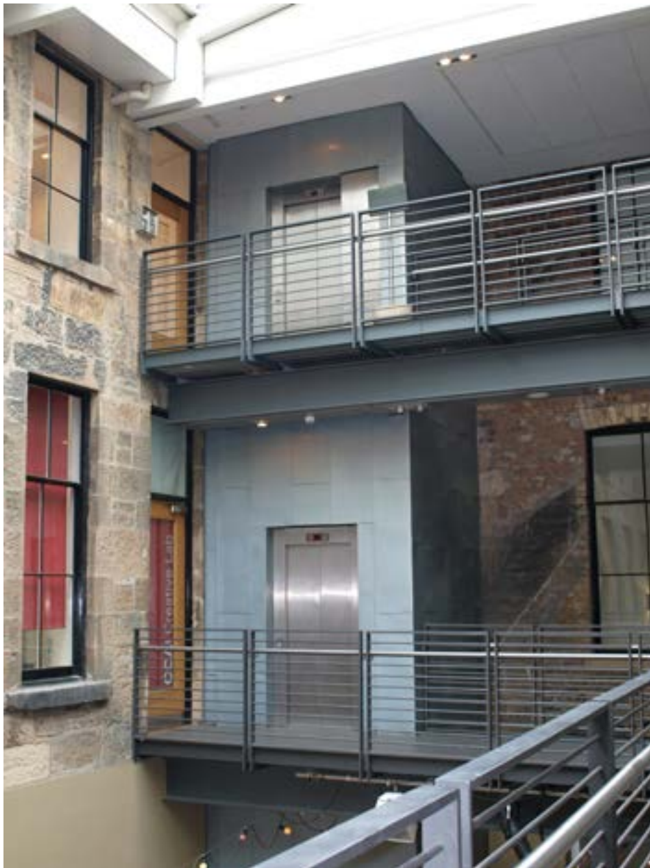
Lift between first and second floor
