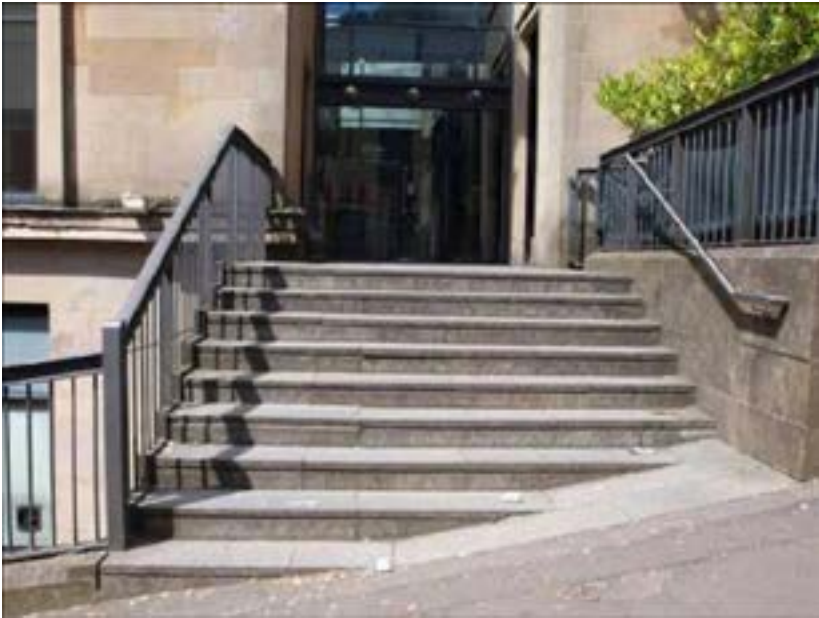
Stairway to entrance from Scott Street
