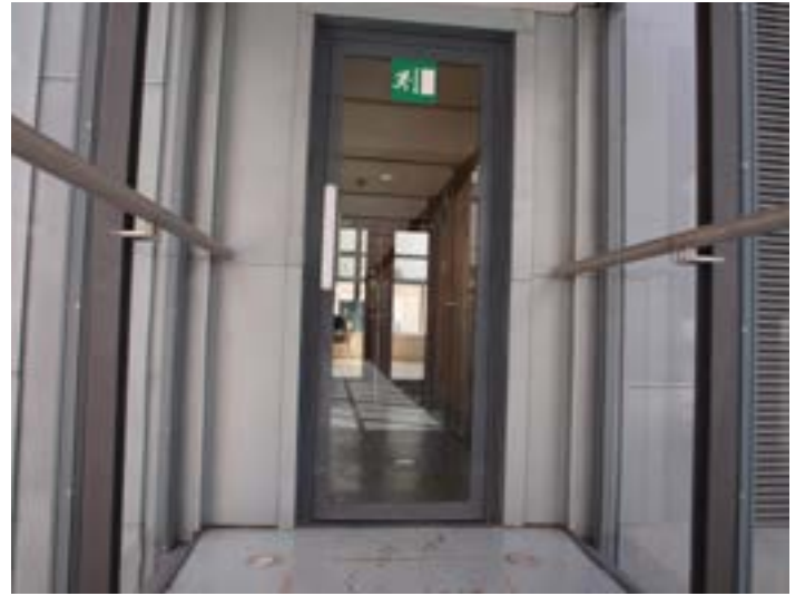
Doorway access to the clubroom
