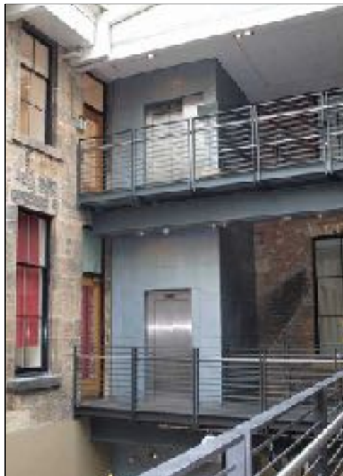
Lift between first and second floor
