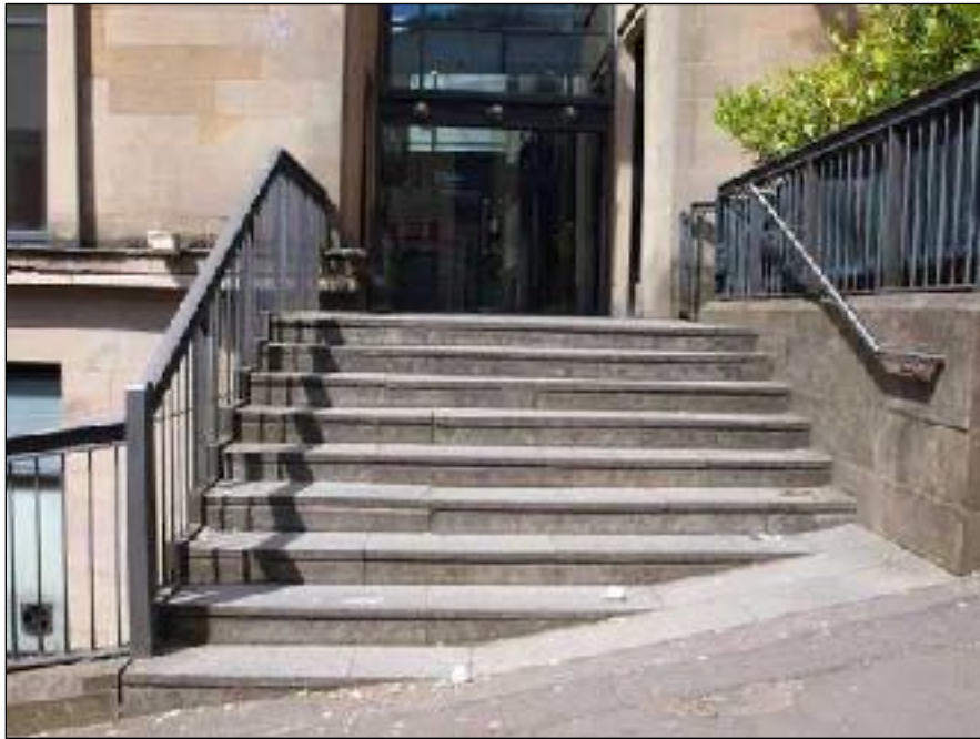
Stairway to entrance from Scott Street
