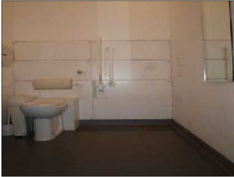
Accessible toilet on first floor
