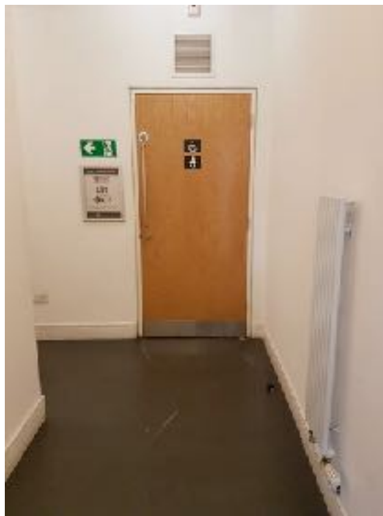
Corridor entry for first floor accessible toilet
