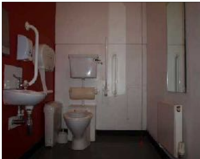
Accessible toilet on ground floor.
