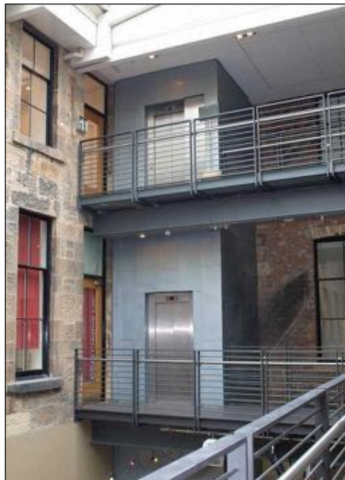
Lift between first and second floor
