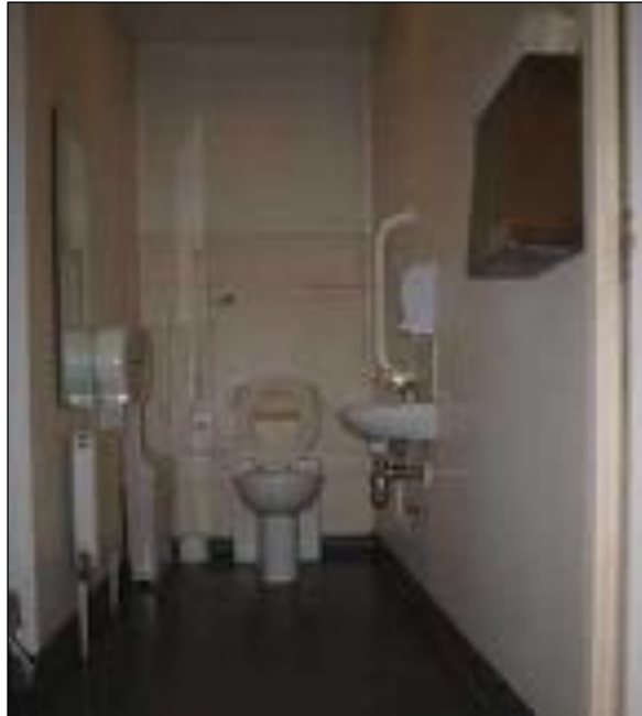
Accessible toilet on second floor
