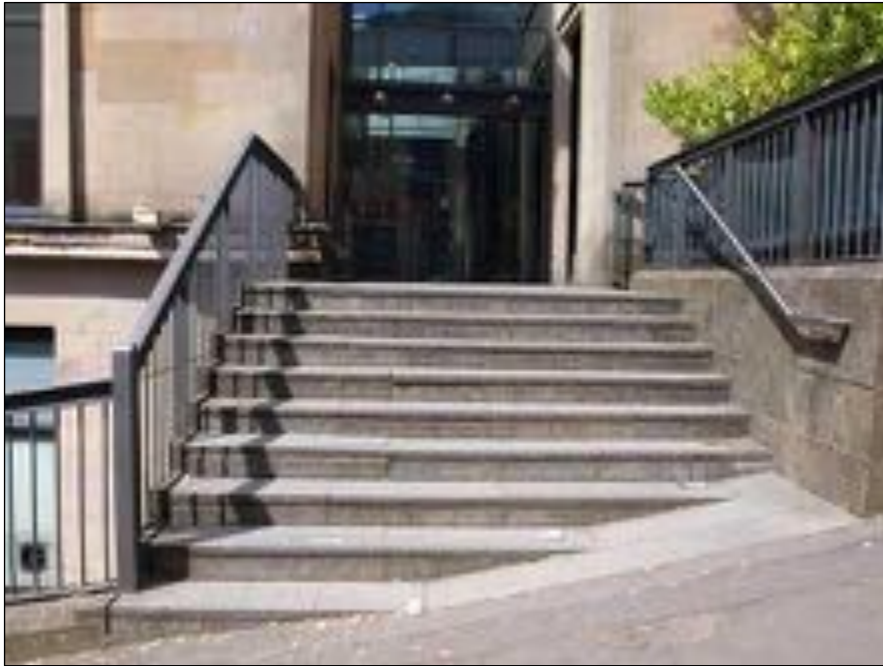
Stairway to entrance from Scott Street
