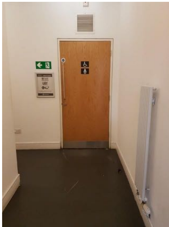
Corridor entry for first floor accessible toilet
