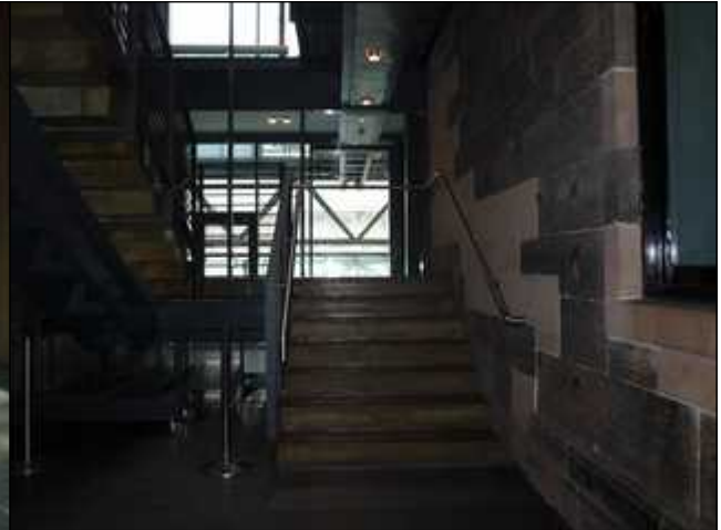
Stairwell from First Floor
