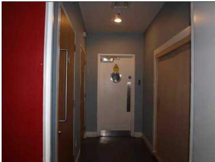
Corridor for ground floor accessible toilets – entrance by bar
